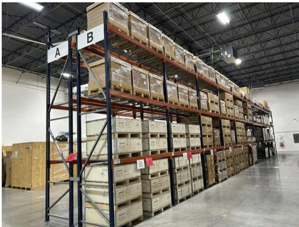
Figure 1: General Storage Conditions
