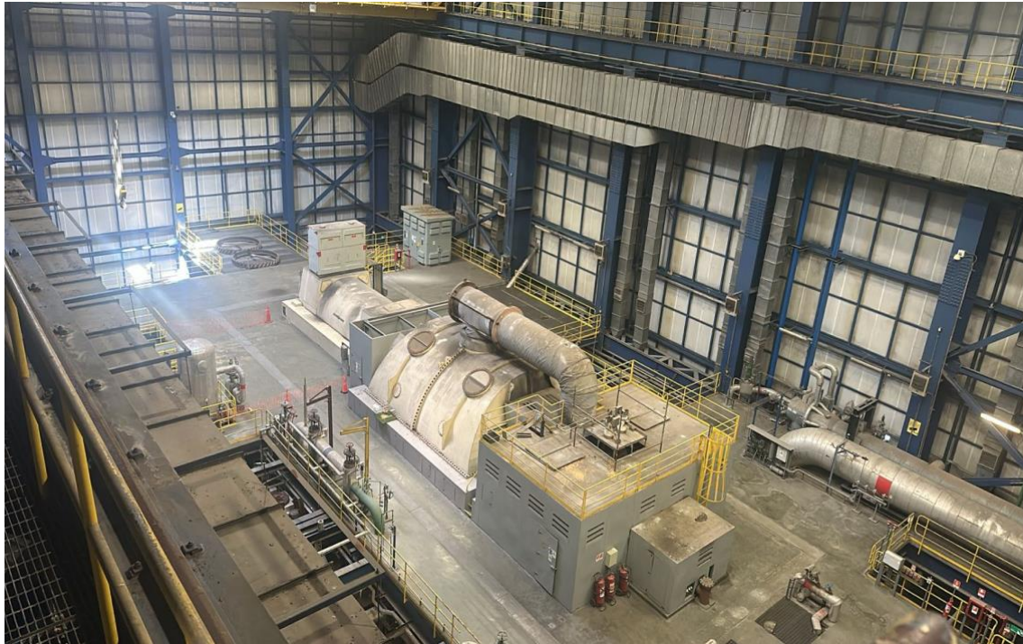
Overview of the steam turbine. In the middle the HP and IP turbine enclosure, left of it the double flow LP turbine followed by the generator with its auxiliaries.
